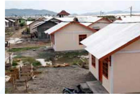
New Housing units in Aceh © UN-HABITAT
